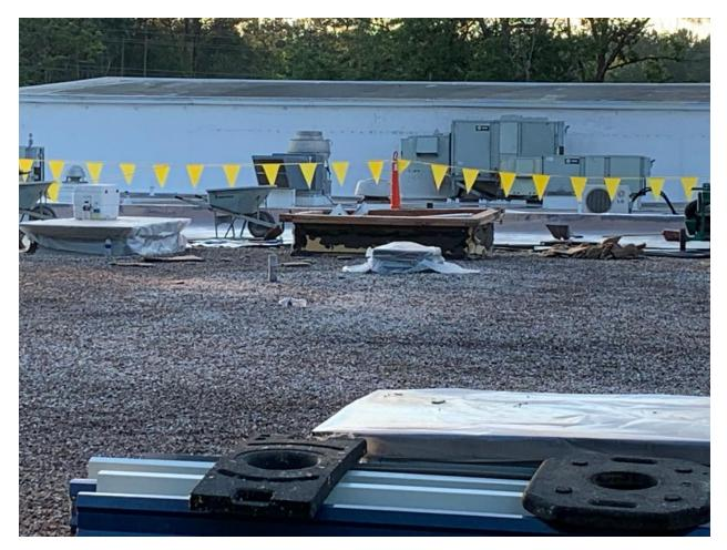
I expect the roof to look considerably different when finished than it did before. All the HVAC equipment will be below the roof. The roof will be built up as much as a foot causing it to drain instead of pooling water and there should be no ballast rock on it to hold it down. This roof had drains we should no longer need shown in previous newsletters. We expect it will be a much better roof system than what we are replacing.
