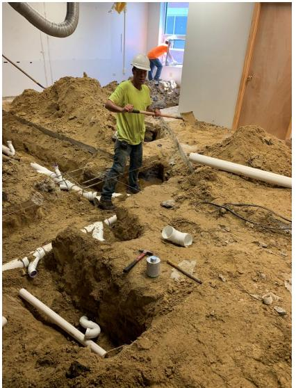
Notice to the left (our right) of the man in the yellow shirt are two old foundations they have tunneled under to route the piping. This is tough work especially in this area with the hot muggy weather AND the insulation is off the metal deck overhead making this area really hot. As we moved through the school the tile with asbestos containing mastic has been removed and the floors are ready for the installation of new tile.
